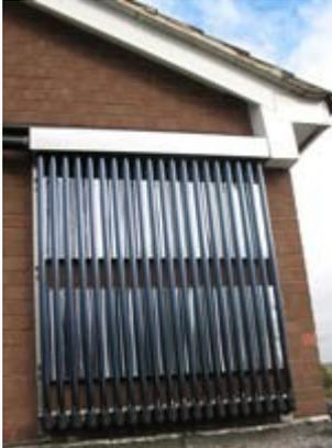
One of the benefits of Evacuated tube panels over simple 'Flat Panels' is that only the frame needs to be assembled in order to mount the panel in its final position. Most of a panel's weight is in the heat pipe assemblies, and these are only fitted once the frame has been secured and the plumbing circuit connected.
